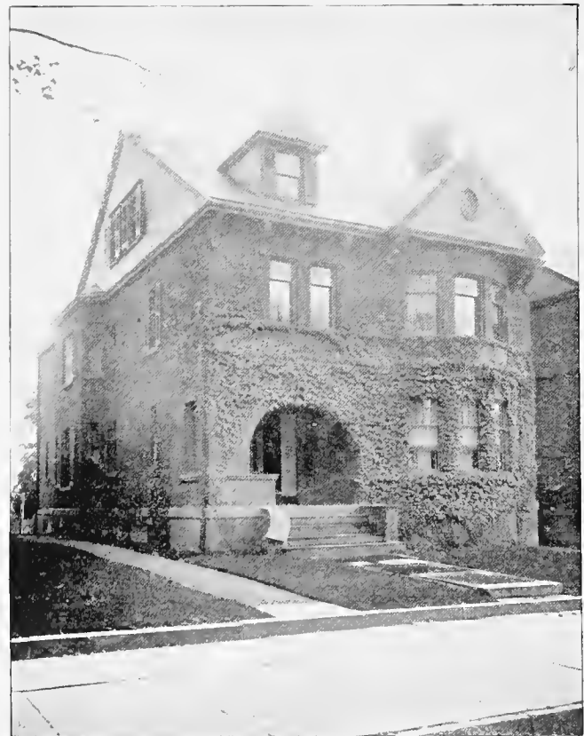
RESIDENCE OF ISAAC C. CHAPMAN—164 Grand Street.
